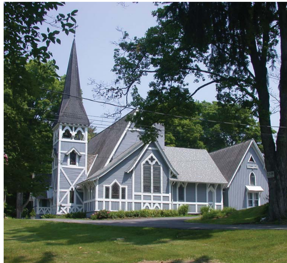
The failing asbestos shingle roof at St. John the Evangelist in Barrytown was replaced at a cost of over $100,000.
